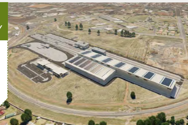
Maintenance facilities in the Dubbo regional railway, in New South Wales (Australia).
