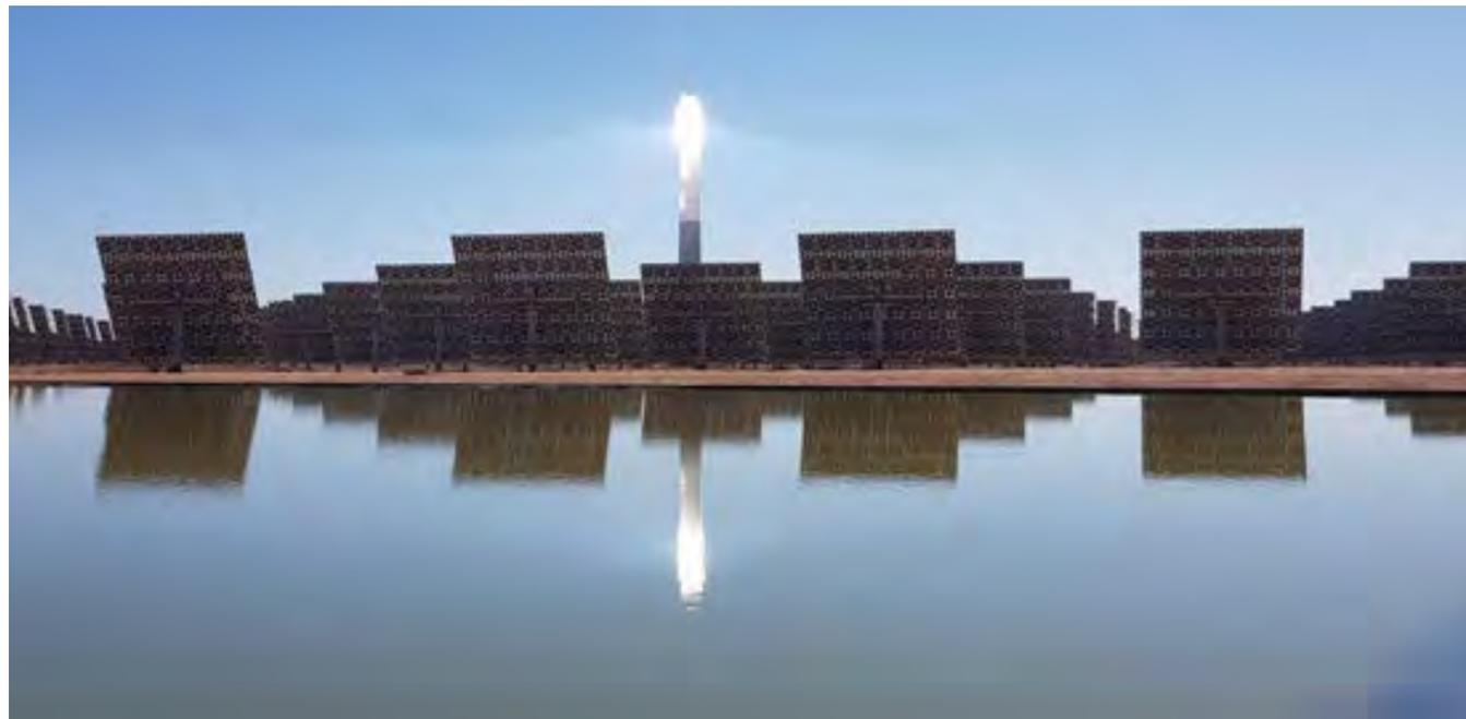
Noor Ouarzazate III solar thermal power plant with central receiver technology and molten salt storage system.
